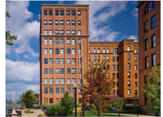
Figure II-2: The Cork Factory Provides Luxury Apartment Living in the Strip District
