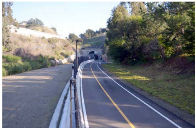
SMART Rail corridor, pre-project build out, with future rail right-of-way and bicycle corridor
