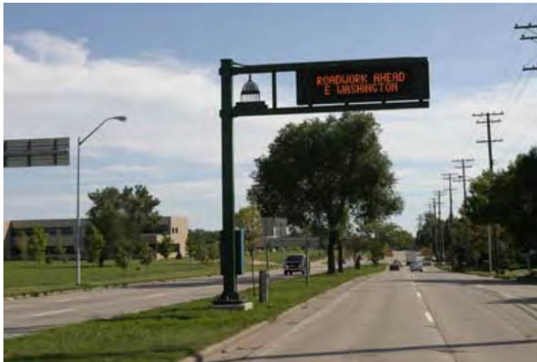
Figure 1.2: Roadside Dynamic Message Signs
