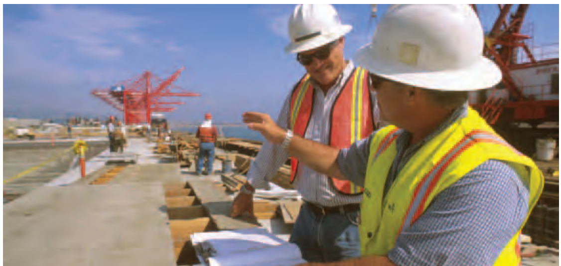
Construction at the Port of Long Beach.
