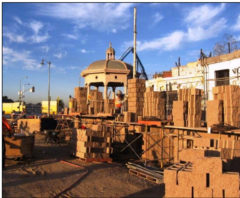
FIGURE 4 Mariachi Plaza Station during construction.
