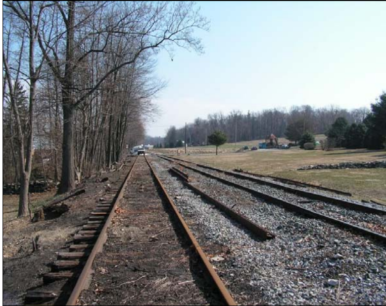
FIGURE 7 Test site near Gettysburg.
