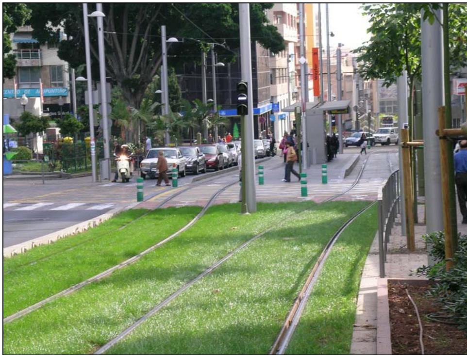
FIGURE 5 Station in which tangent tract is not extended to both sides of the platform, Tenerife light rail.
