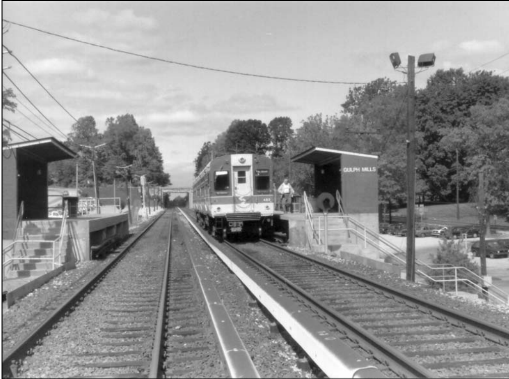
FIGURE 9 CTA “L” car at Gulph Mills Station.
