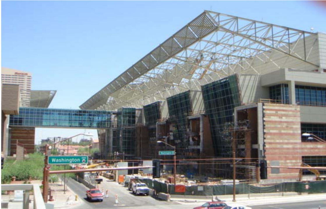
FIGURE 7 Phoenix Convention Center (foreground) and Sheraton Phoenix Downtown (background, left).
