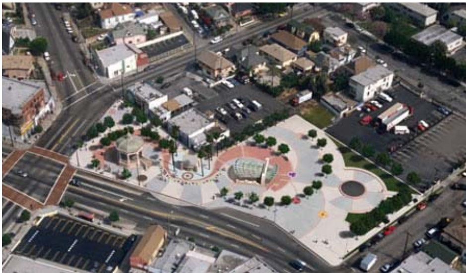
FIGURE 2 Aerial view of Boyle Heights–Mariachi Plaza Station at 1st Street and Boyle Avenue.
