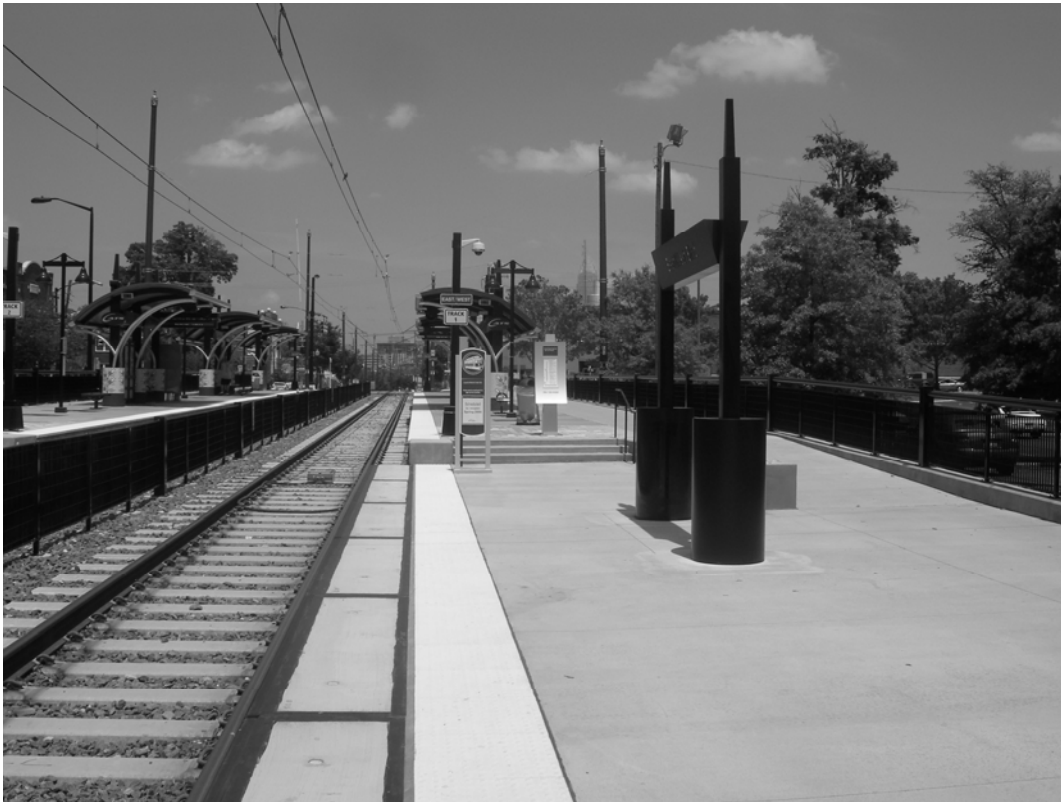
FIGURE 1 Light rail and replica trolleys have separate but adjacent platforms in Charlotte. The trolley boarding area is at the front of the above picture, and the raised light rail platform is in the rear.
