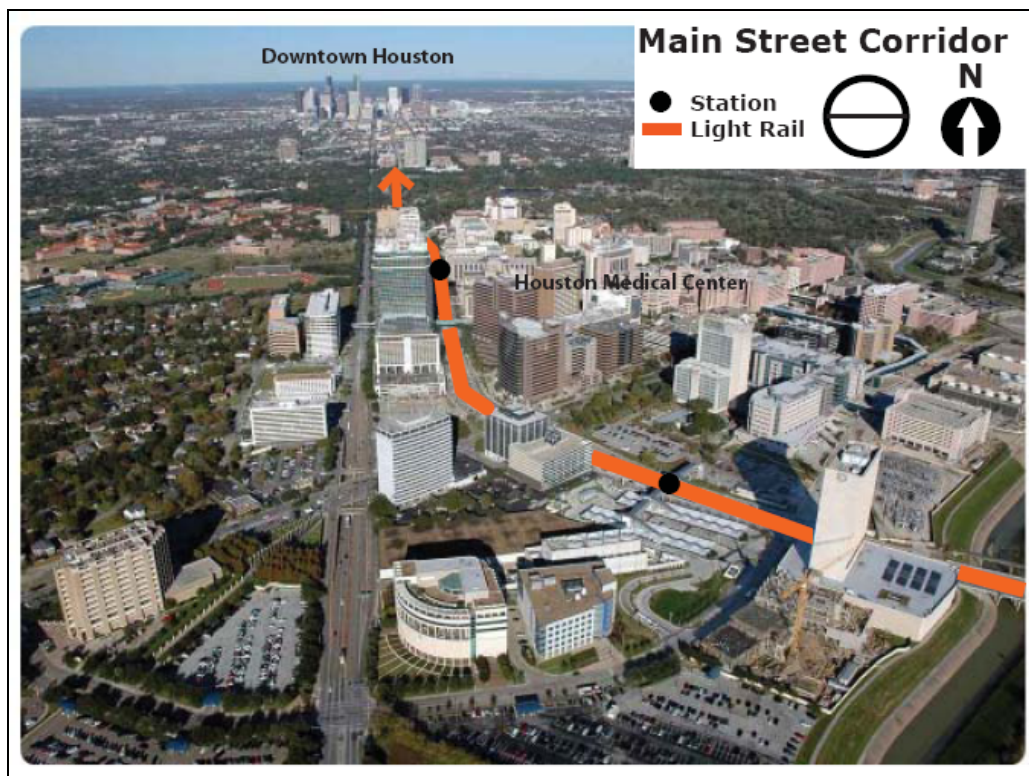
FIGURE 4 Houston light rail in the medical center.
