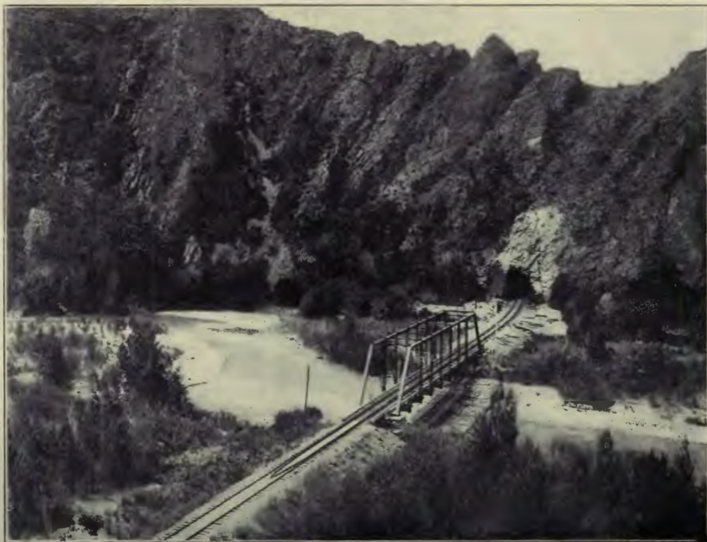
TUNNEL NO. 3, WEBER CANYON, ON UNION PACIFIC RAILWAY
