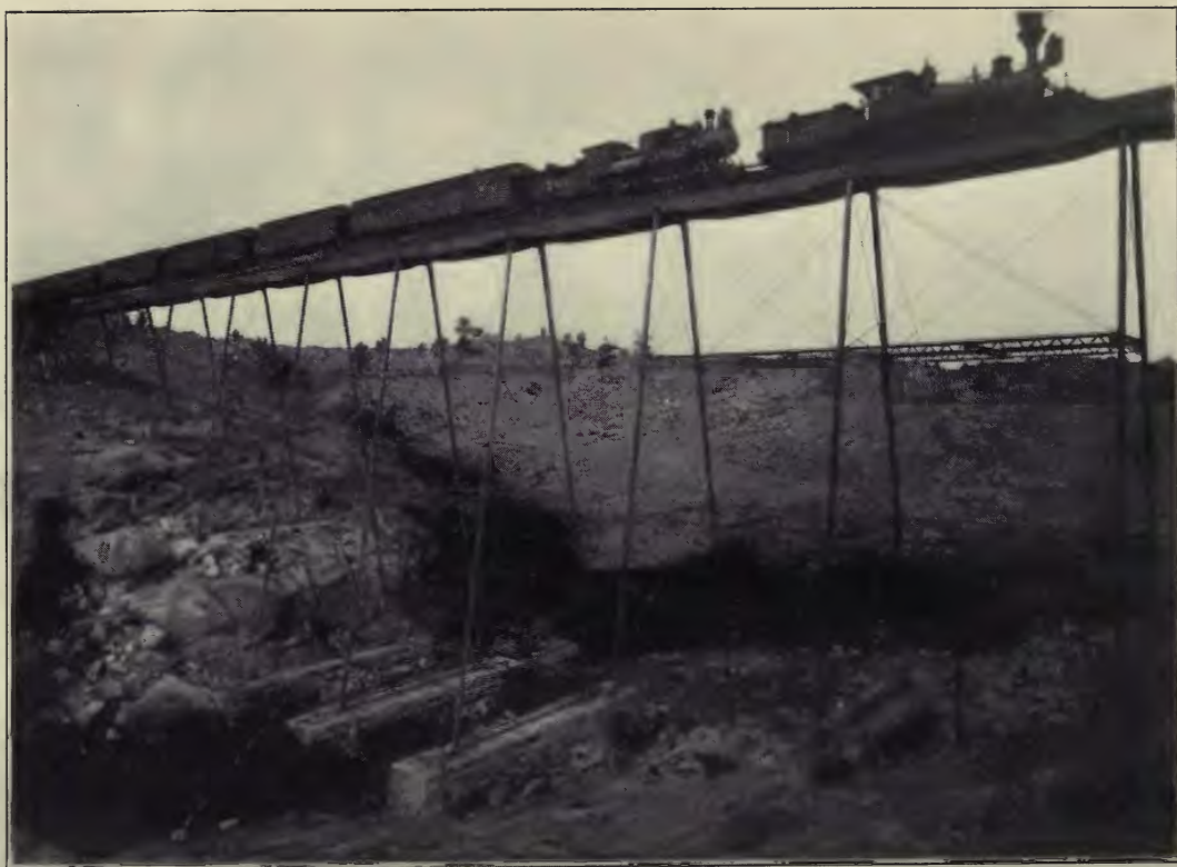
DALE CREEK BRIDGE Main Line, Union Pacific Railway
