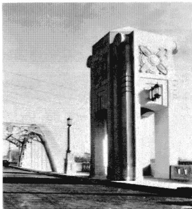
5 th Street bridge over the Los Angeles River
