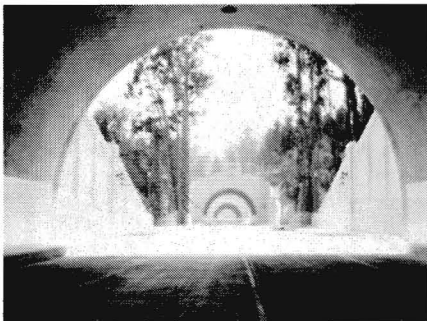
The original three Figueroa Street tunnels in 1931.
