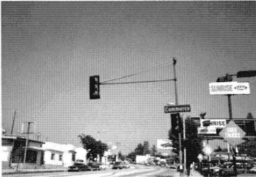
1946 mastarm at Foothill Boulevard and Commerce Avenue Graphic - 3110
