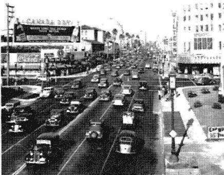
Wilshire Boulevard at Western Avenue, 1937 Graphic—5037
