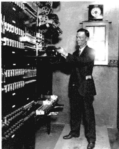
Acme Signal Center in Pershing Square basement, circa 1924 Graphic - 3080
