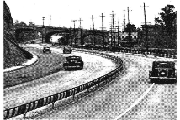
Ramona Parkway at the Macy Street Overcrossing, showing the special guard rail Graphic - 8090
