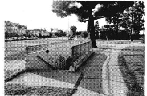
Crescent Heights Boulevard pedestrian tunnel under Olympic Boulevard Graphic - 2054
