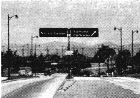
Modern "butterfly" sign versus the traditional Auto Club sign on the Santa Ana Freeway at Ramona Parkway (San Bernardino Freeway), 1949 Graphic - 8111
