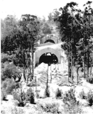
Construction of the Figueroa Street tunnels
