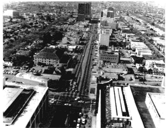
Southern California's first Two-Way Turn Lane in May 1960 on Wilshire Boulevard, easterly of Fairfax Avenue. Graphic 3104
