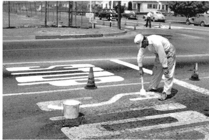
Pavement message maintenance using a brush, circa 1950
