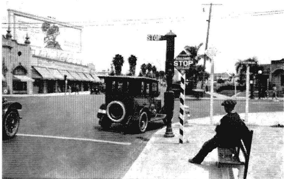
The second Acme signal style, circa 1926, on Wilshire Boulevard at Western Avenue Graphic - 1021
