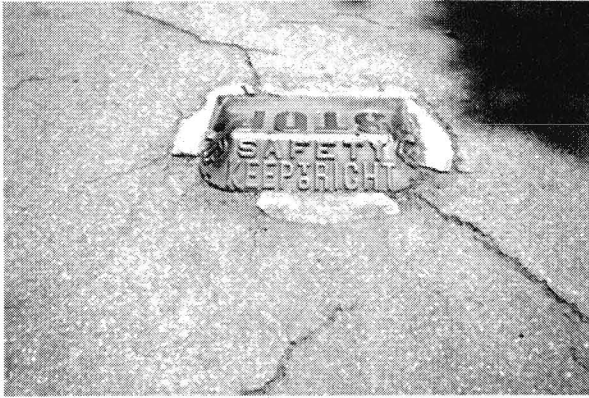
Metal pavement marking from the 1920's
