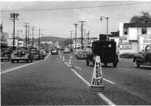
Reversible lane operation along Figueroa Street, south of Sunset Boulevard, looking north, circa 1949 Graphics - 3011
