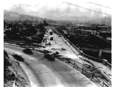
Construction of the Figueroa Street bridge over the Los Angeles River.
