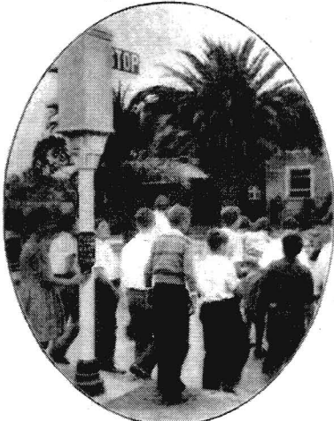
Pedestrians can now act as their own traffic officers with the invention of a new street crossing device by Ralph Dorsey, Los Angeles traffic signal engineer, which is now being tried out. Operated by a push-button, this work-it-yourself signal halts traffic with stop arms and red light for 15 seconds, giving the pedestrians time to cross the street, then it automatically reverts to the "clear" position. Twenty-five seconds must then elapse before another pedestrian can again halt traffic. Photo shows pupils from the Luther Burbank Junior High School in Los Angeles operating the new device.
