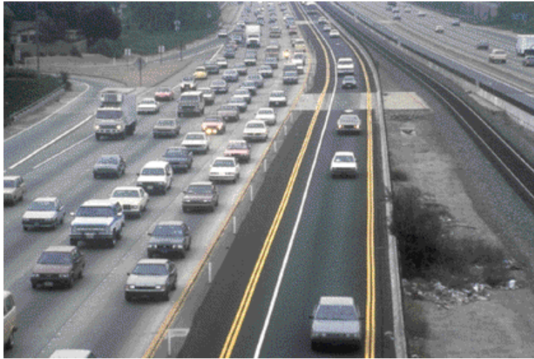
Figure 3. El Monte Busway Buffer Separated Section
