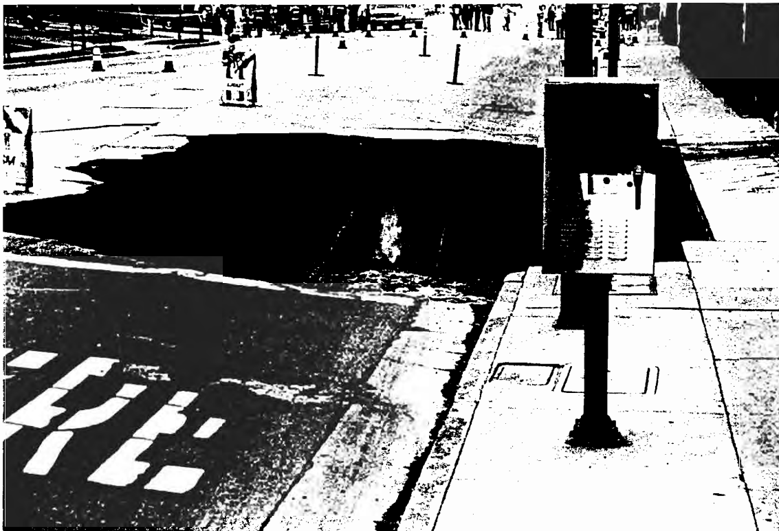
Fig. 2.4 - Water main pouring into sinkhole above tunnel collapse
