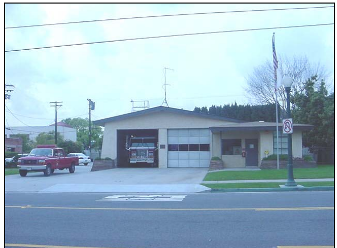
Fire Station 52 is the smaller of the two fire stations. Its bays will soon be too small to hold state-of-the-art fire trucks.
