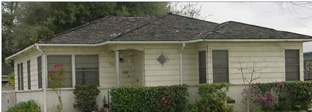
Single-family homes still account for over 60% of the city's total housing stock.
