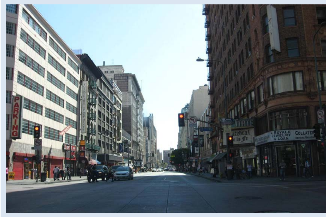
Photo 5. Broadway at West 7 th Street, Looking South
