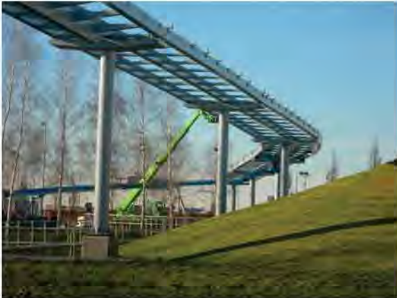
Elevated carriageway is light weight and easy to construct using off-site prefabricated elements.
