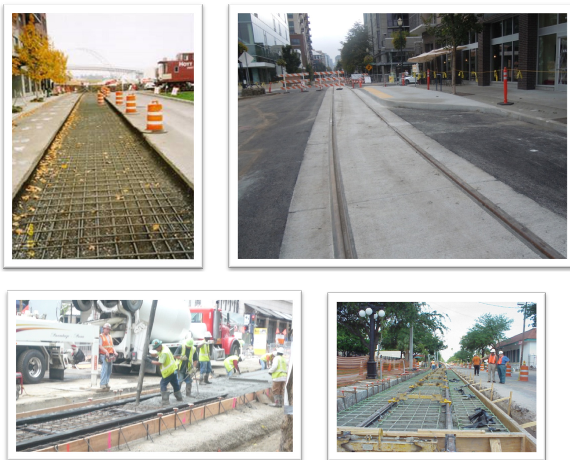
Figure 3-2 Streetcar Trackwork Construction (Portland, OR)
