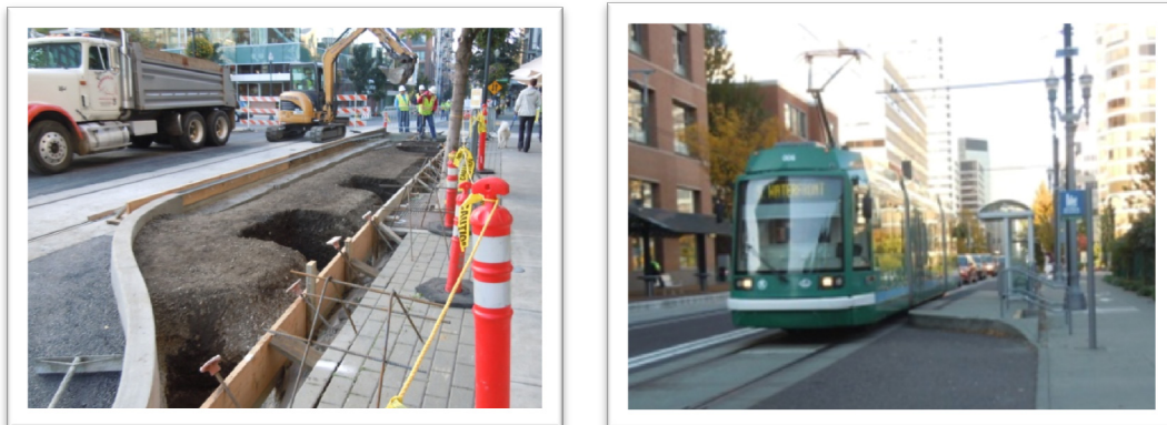
Figure 3-3 Streetcar Stop Platform Construction (Portland, OR)
