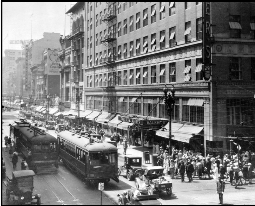
Looking South down Broadway at the Intersection of 5 th Street in 1926. Streetcars Proceed down the Center of Broadway.
