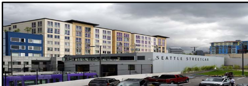
Seattle South Lake Union Streetcar Maintenance and Storage Facility (HDR 2013)
