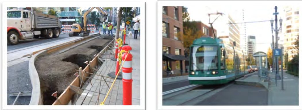
Figure 3-3 Streetcar Stop Platform Construction (Portland, OR)
