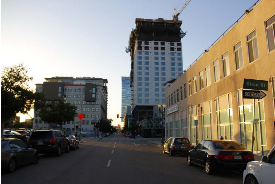
Figure 3.1-7. West 11 th Street, Approaching Olive Street, Looking West
