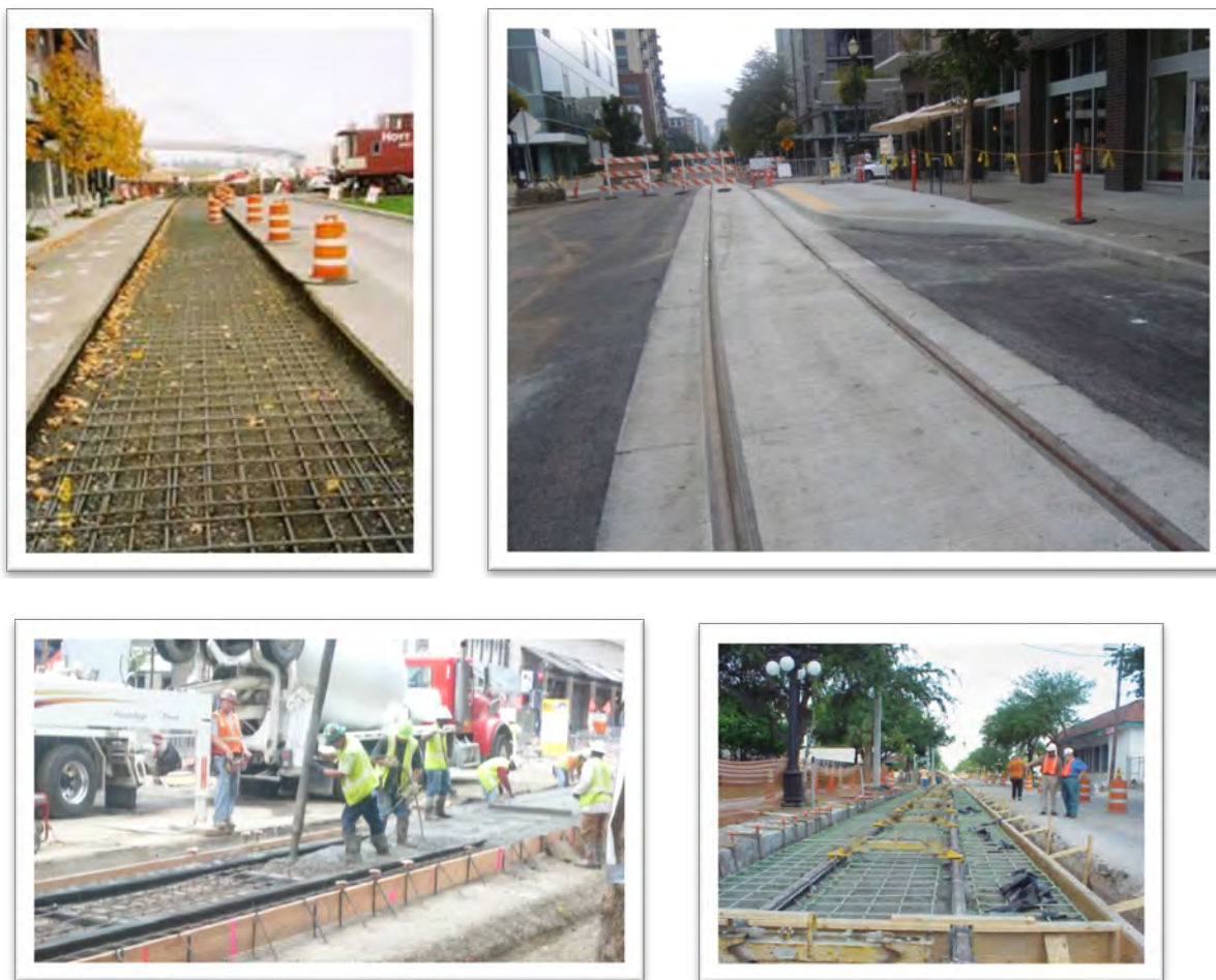
Figure 3-2 Streetcar Trackwork Construction (Portland, OR)
