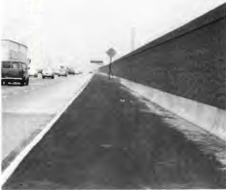
Soundwalls reduce freeway noise.
