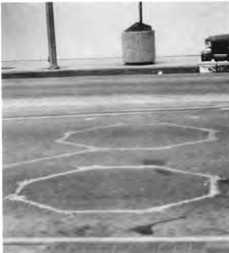
Cars are counted by loop detectors.
