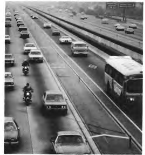
The El Monte Busway moves more people than any one of the adjacent freeway lanes.
