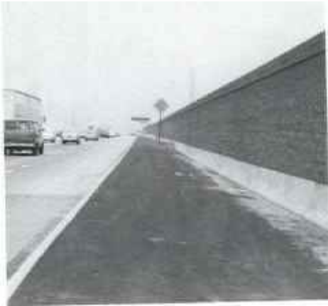
Soundwalls reduce freeway noise.
