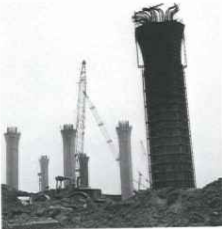
Construction of the Century Freeway in progress.
