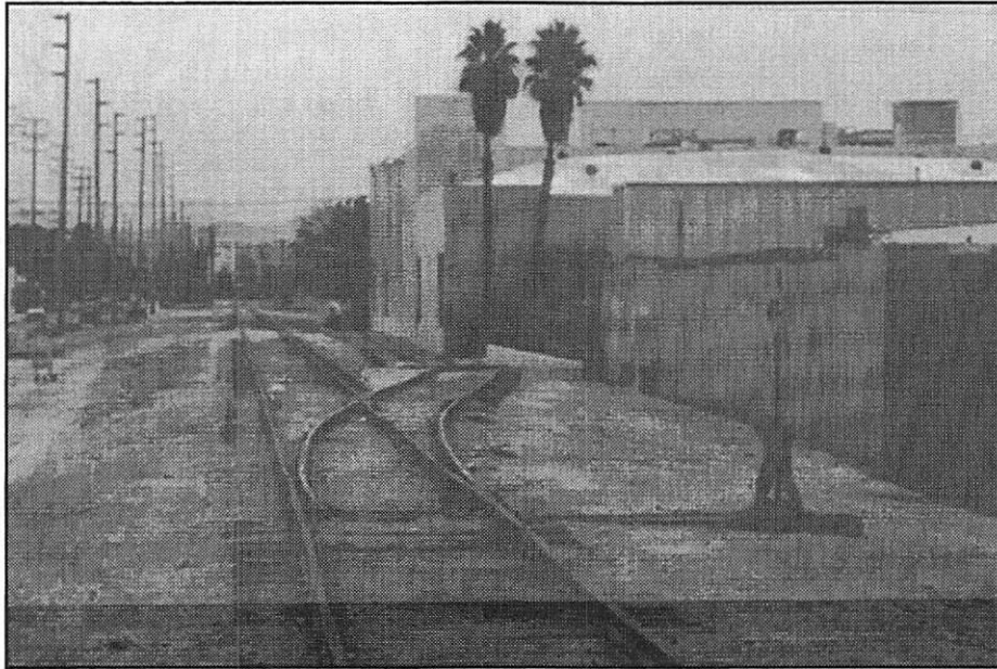
The SP right-of-way in an industrial area within the Los Angeles city limits, near Cahuenga Boulevard.
