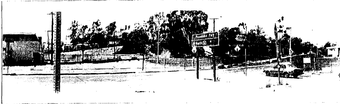
Route B1: At the intersection of Bernard Street and the Pasadena Freeway, the elevated guideway would turn to follow the northbound Dodger Stadium off-ramp, seen at the right of the photo. The guideway would climb at a 6% to 10% grade in order to gain 225 feet of elevation between North Broadway and Dodger Stadium.
