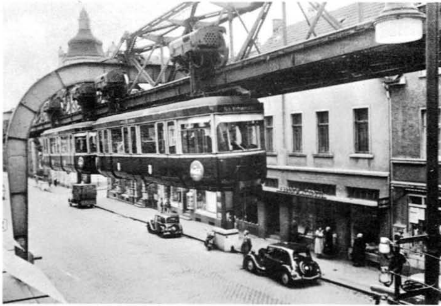
CLASSICAL MONORAIL - SUSPENDED ASYMMETRICAL View of Monorail Operating in Wuppertal, Germany Since 1903
