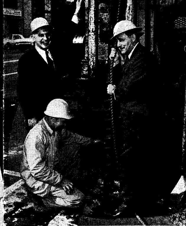
TWO WEEKS LATER (Jan. 23) drilling begins in the Beverly Hills area at Linden Dr. and Wilshire Blvd. Here Driller Bill Schwenk is "assisted" by N. R. Dumont, MTA Board member, left; and Jack Freeman, Mayor of Beverly Hills, right.
