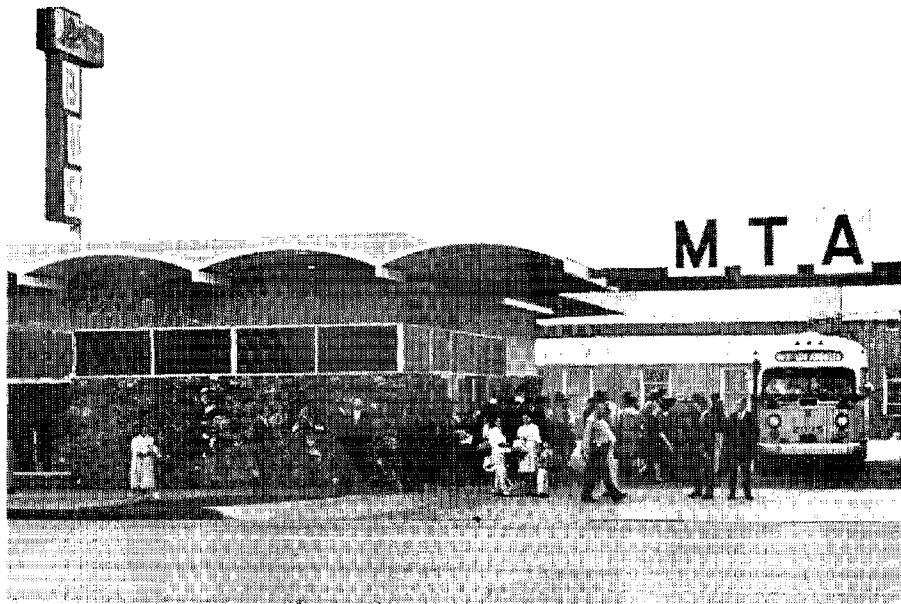
TYPICAL SUBURBAN STATION AT RIVERSIDE
