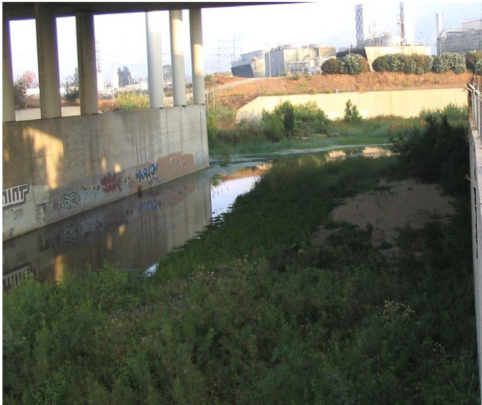
Figure 3.7-5 Verdugo Wash at the Confluence with the Los Angeles River
