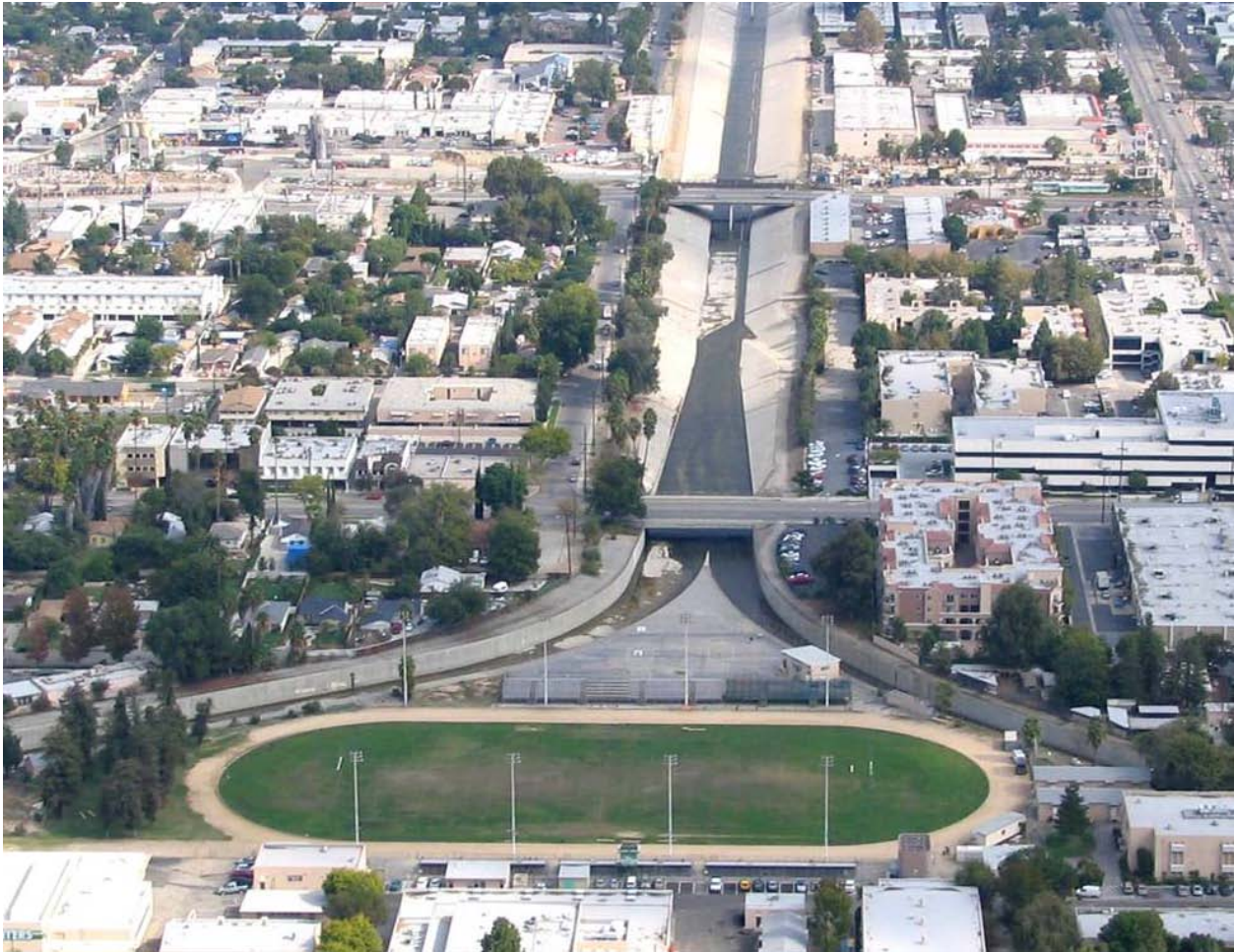
Figure 3.5-1 Channelized portions of Arroyo Calabasas and Bell Creek converging to form the Los Angeles River at Canoga Park High School
