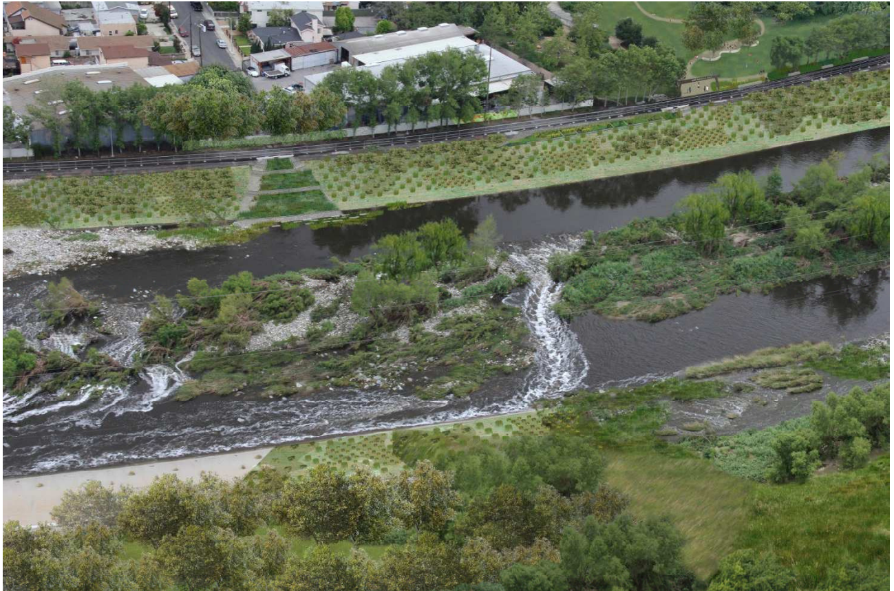
Figure 4-26. Reach 6. Looking West, with the Bowtie Parcel in the Foreground and Marsh Park in the Background. Existing Channel and Rendering of Proposed Daylighted Stream and Vegetated Walls.
