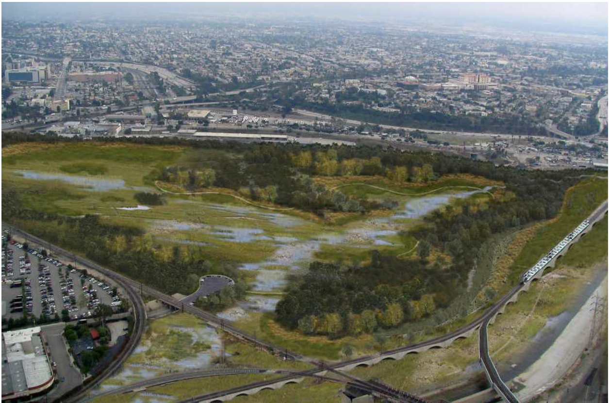
Figure 4-30. Reach 8. Piggyback Yard, Looking Southeastward Existing and Rendering of Proposed Restoration Measures
