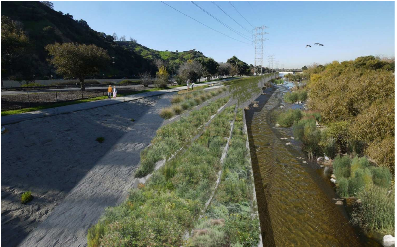
Figure 4-22. Reach 2. Looking Upstream from Riverside Drive Bridge Existing Channel and Rendering of Proposed Terraced Banks/Vegetated Channel Walls
