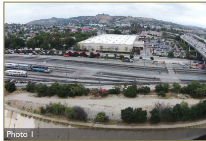
Top of bank area South of SR-110, looking West.
