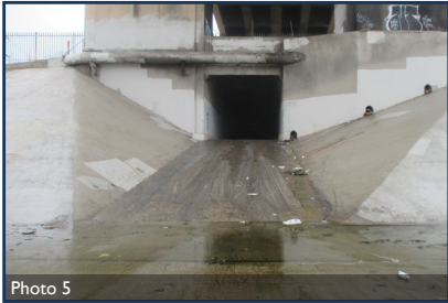
Location of existing maintenance access tunnel at 6th Street, looking West.
