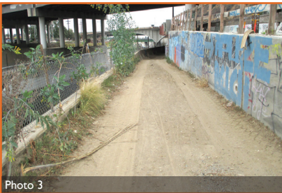
Top of bank area. Looking South under I-5 overpass.
