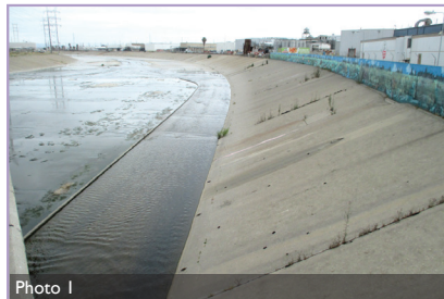
Photo 1 Channel wall area South of Bandini Boulevard, looking South.
