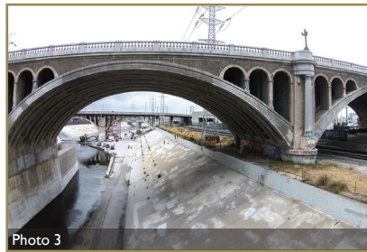
Looking South under historic Broadway Bridge.
