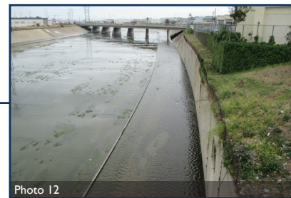
Looking South at Bandini Street Bridge.
