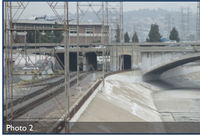
Looking North at the US-101 freeway.
