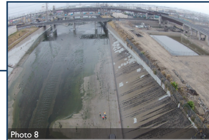
Looking South at Washington Boulevard Bridge and railroad crossings.
