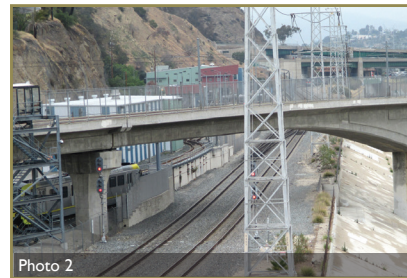
Top of bank area at Metro railroad crossing North of Broadway, looking North.
