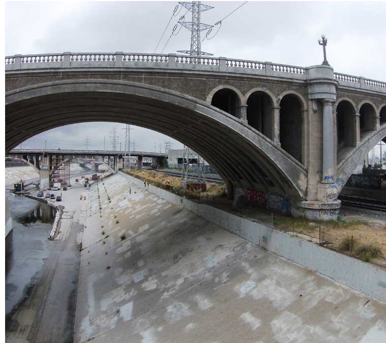
Figure 2-1: Photo of historical Broadway Bridge
