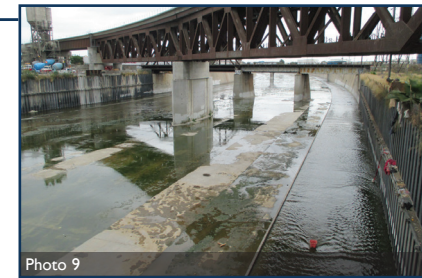
Channel bottom area South of Washington Boulevard, looking South.
