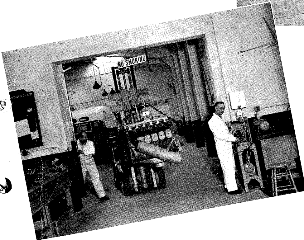
● Clark Lift rolls motor from the unit overhaul department to the installation section.
