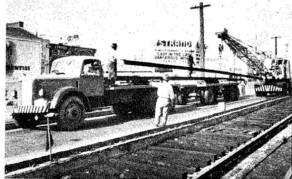
Rubber mounted crane replaces rails without blocking streetcar traffic.
