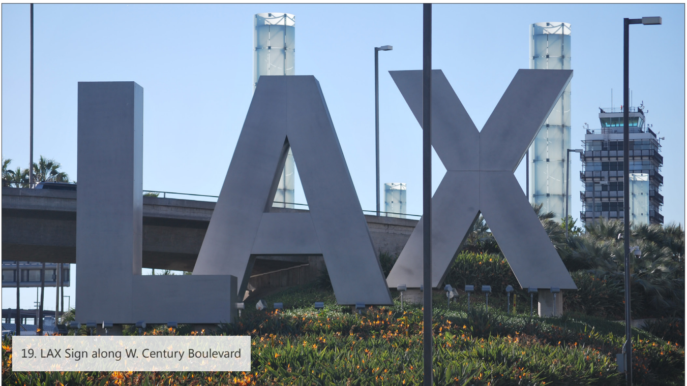
18. LAX Airport Entrance Interchange Illuminated Pylons (as viewed from the west)
