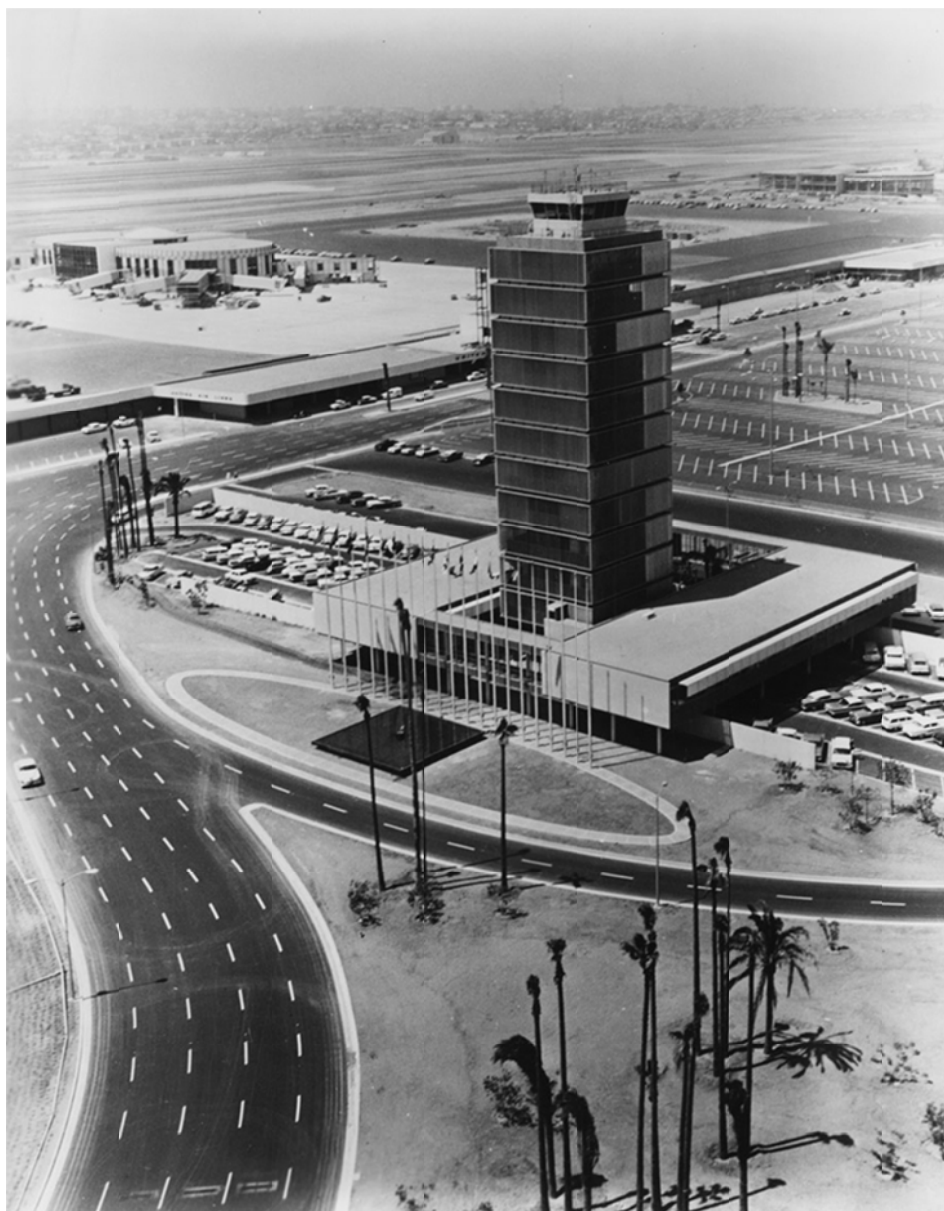
Central Terminal Completed 1961 Los Angeles Water & Power Collection
