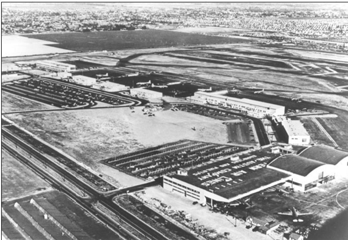
Los Angeles International Airport Intermediate Facilities c. 1955
