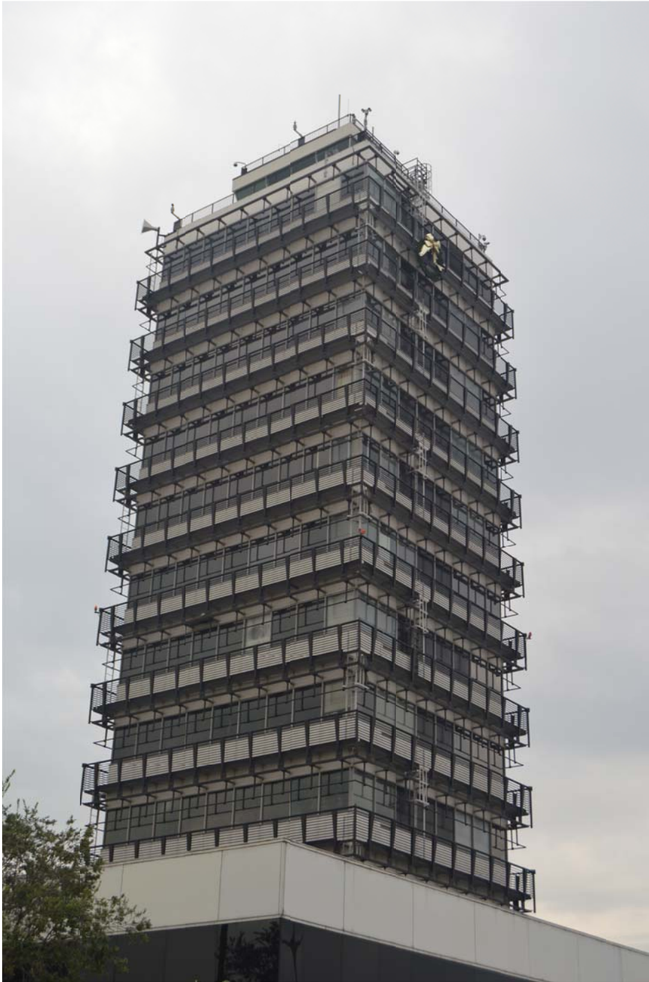
CTA Tower, December 2014
