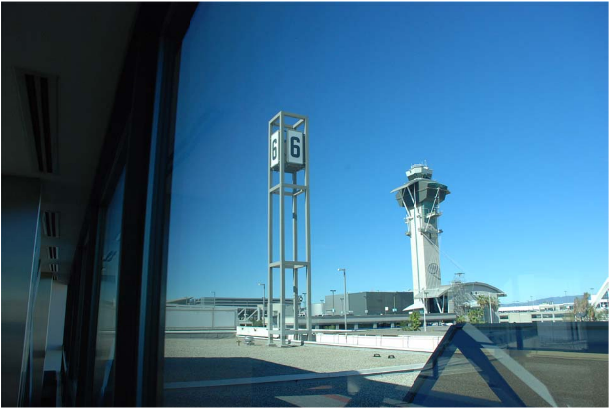
Terminal 6 Pylon, February 2015
