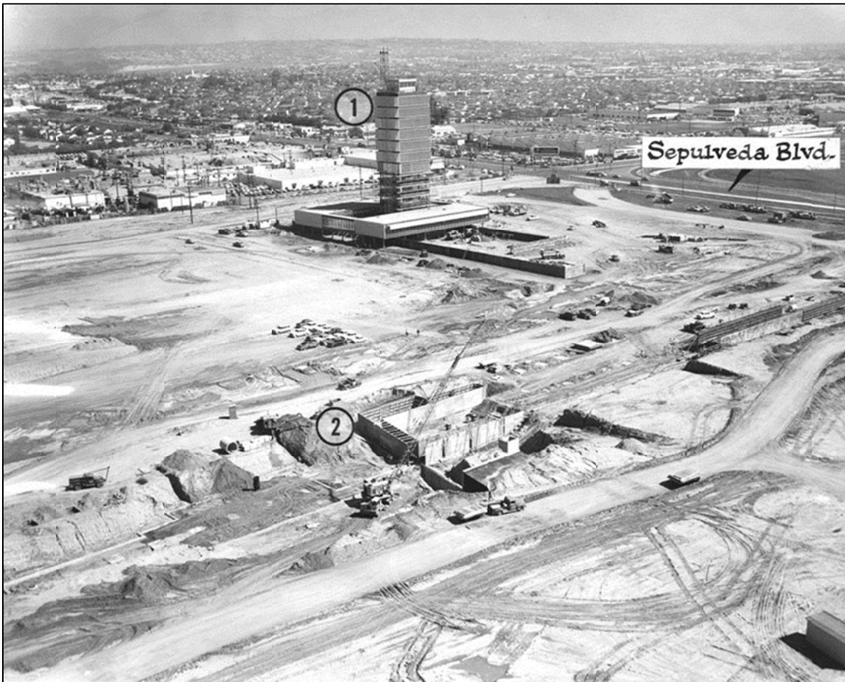
Central Terminal Area Under Construction 1960 Los Angeles Public Library
