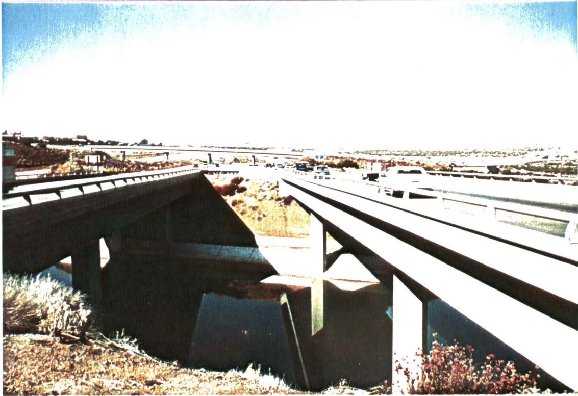
FIGURE 12.20 HOLT TO AVENUE "S" (STATION 12 TO 13) 14 FREEWAY & CALIFORNIA AQUEDUCT - LOOKING NORTH
