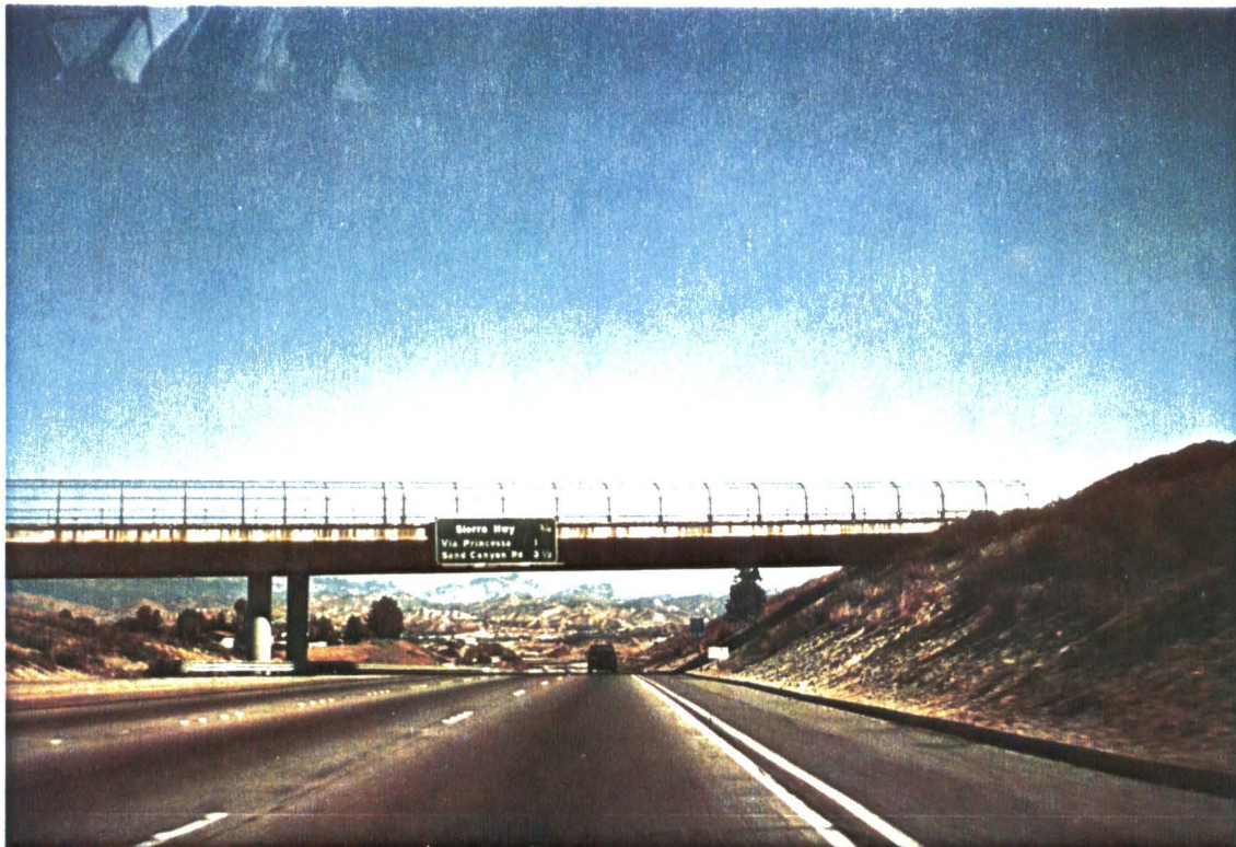
14 FREEWAY & GOLDEN VALLEY OVERPASS - LOOKING NORTH
