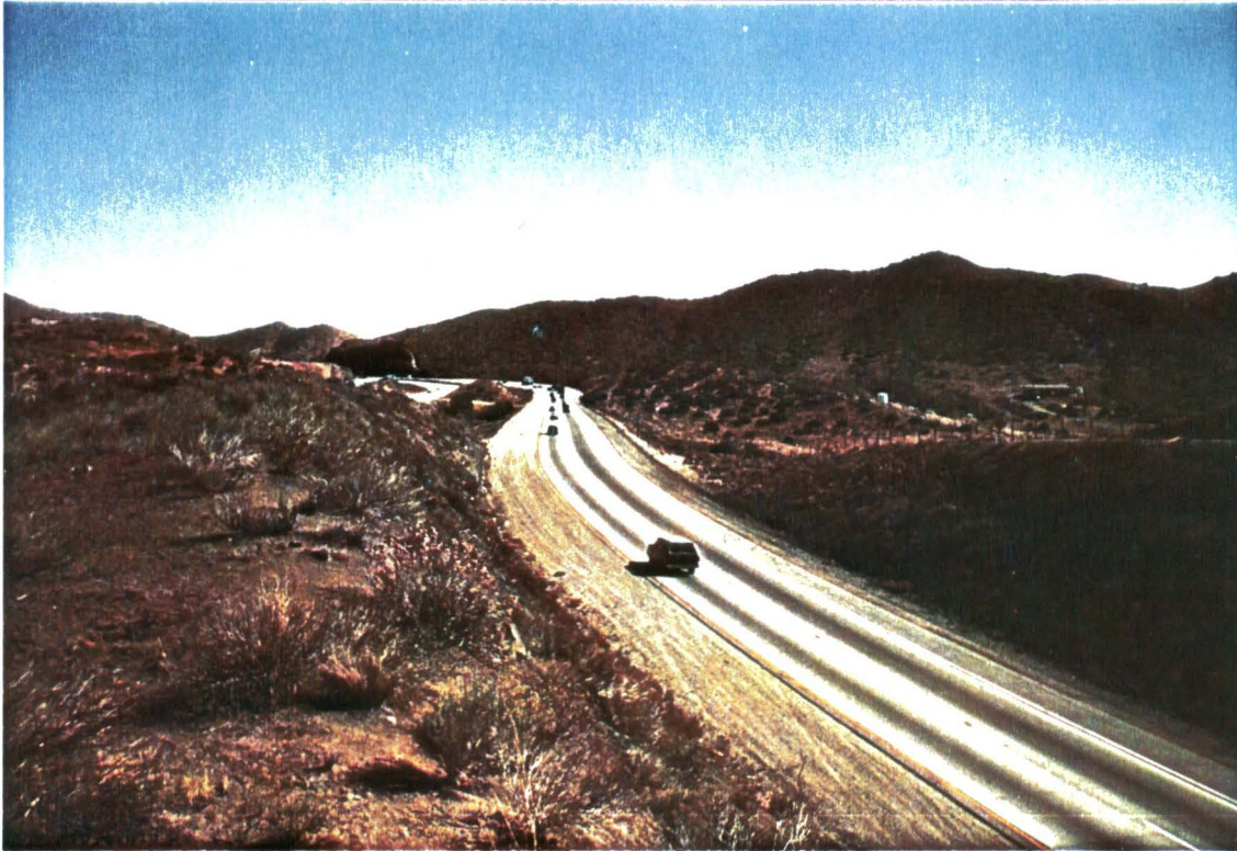
FIGURE 12.19 HOLT TO AVENUE "S" (STATION 12 TO 13) 14 FREEWAY & CROWN VALLEY ROAD - LOOKING WEST
