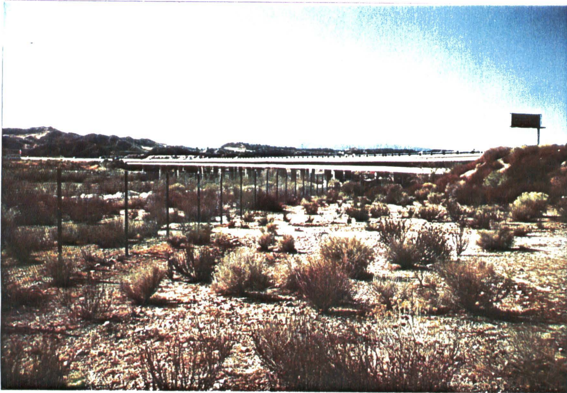
FIGURE 12.16 HOLT TO AVENUE "S" (STATION 12 TO 13) 14 FREEWAY & SANTA CLARA RIVER - LOOKING WEST
