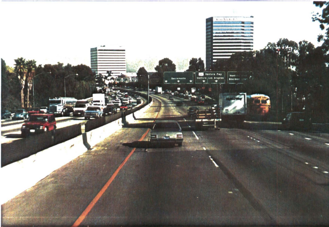
FIGURE 6.2 VENTURA TO VICTORY (STATION 6 TO 7) 405 FREEWAY & 101 FREEWAY - LOOKING NORTH
