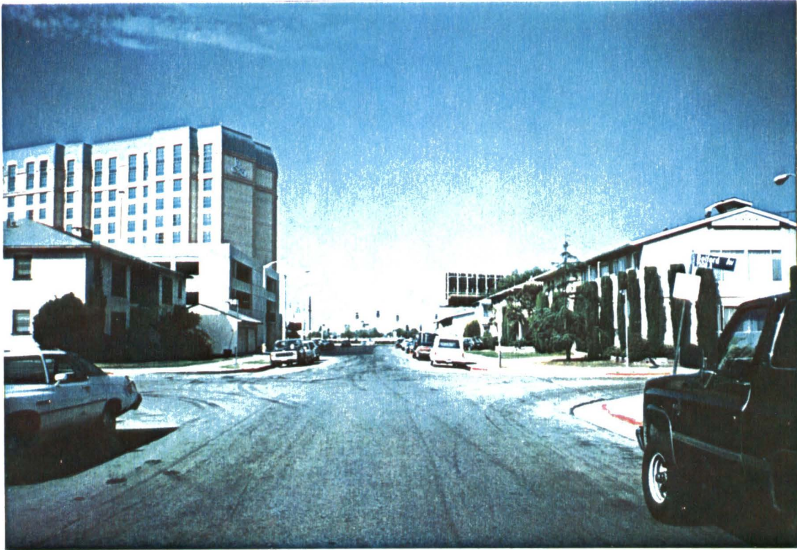
FIGURE 1.4 LAX TO MARINA FREEWAY (STATION 1 TO 2) 96TH STREET & BEDFORD AVENUE - LOOKING WEST
