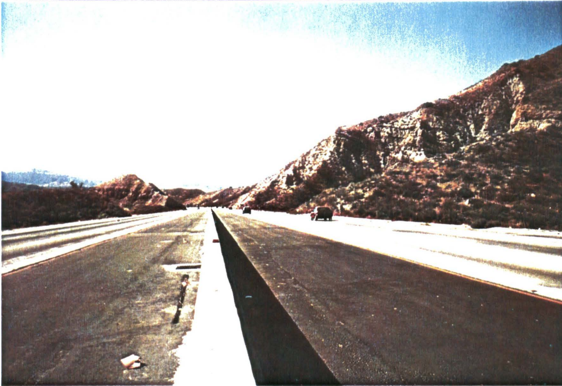
FIGURE 12.17 HOLT TO AVENUE "S" (STATION 12 TO 13) 14 FREEWAY & SPRING CANYON ROAD - LOOKING SOUTH
