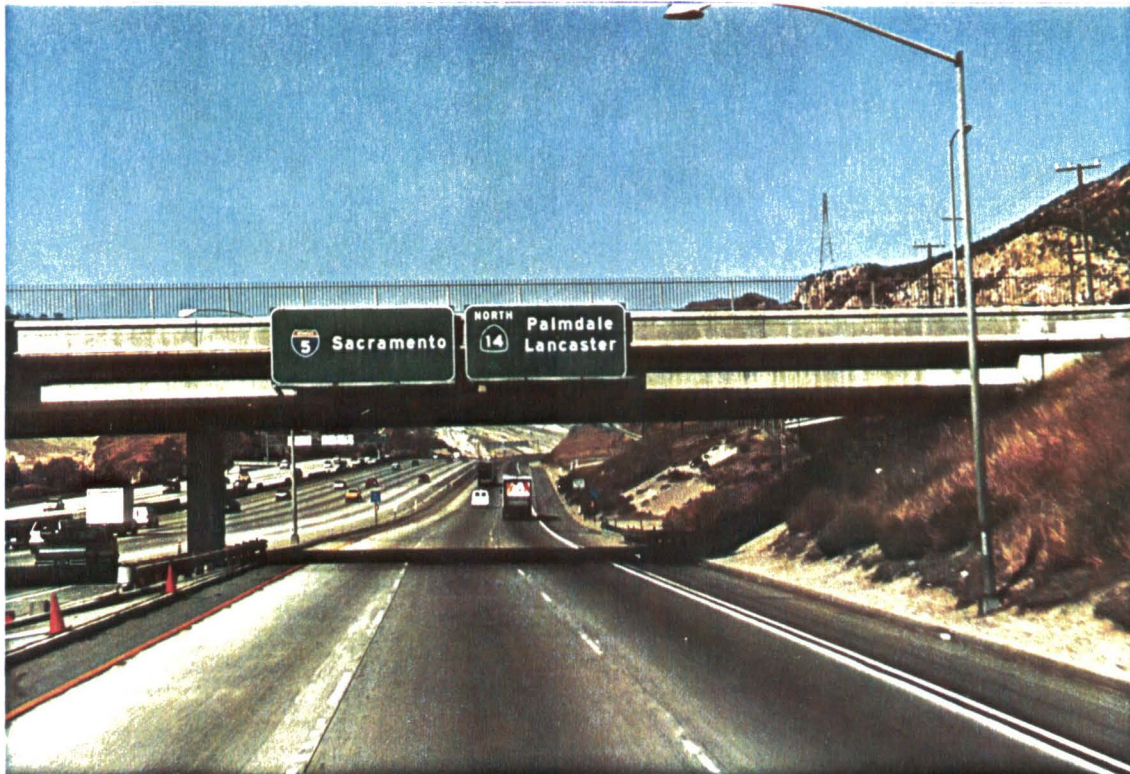
5 FREEWAY & BALBOA BRIDGE - LOOKING NORTHWEST
