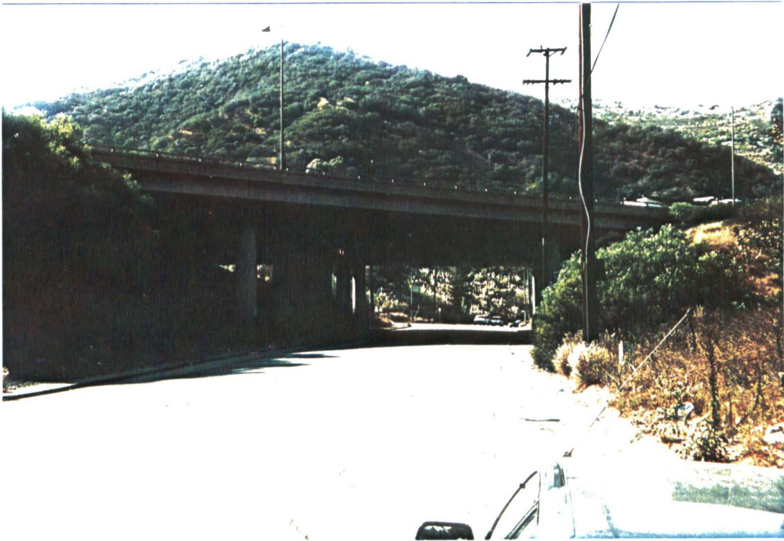
FIGURE 5.7 WILSHIRE TO VENTURA (STATION 5 TO 6) SEPULVEDA BLVD. & 405 FREEWAY - LOOKING WEST
