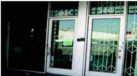
Interior grills that are more than 75% open are less visible during non business hours and easier to screen from view during business hours.
