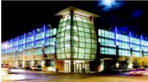
Pre-cast panel and glass louver screening plus photovoltaic panels on top deck (upper), and metal screen with tower element marking the entry corner and vertical circulation (lower).
