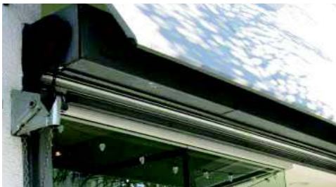
Awnings can be used to conceal existing exterior roll-down doors during business hours.
