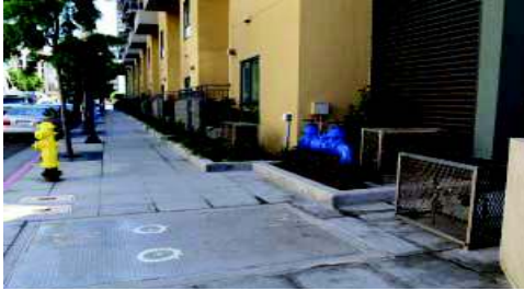
Examples of poor equipment location choices. A primary opening to the courtyard garden is walled off with electric meters and irrigation equipment in plain view near a building entrance.
