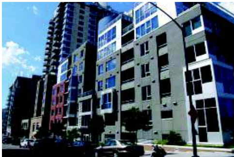
6 - and 7 - story street wall Walls above the ground floor that step back less than 15 feet from the ground floor street wall are part of the street wall, as illustrated above.
