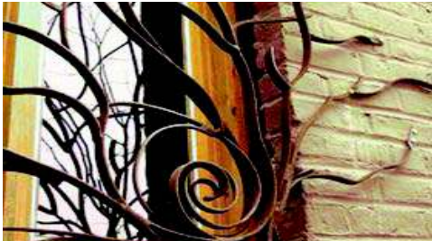
There are always exceptions: this security grill is not retractable, but could be approved given its aesthetic contribution.
