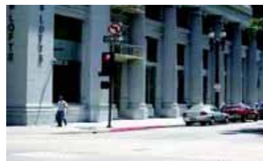
Similarly, columns are at the property line, while the facade is set back a few feet.
