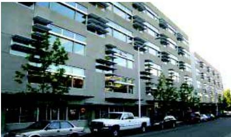
Windows should be well-detailed and have a recessed depth.
