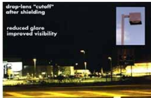
The cinema complex in Branford, Connecticut, before and after its lights were fitted with full cutoff shields to comply with the town's new regulations. The change kept the ground well lit while dramatically reducing glare and light trespass onto neighboring property.
