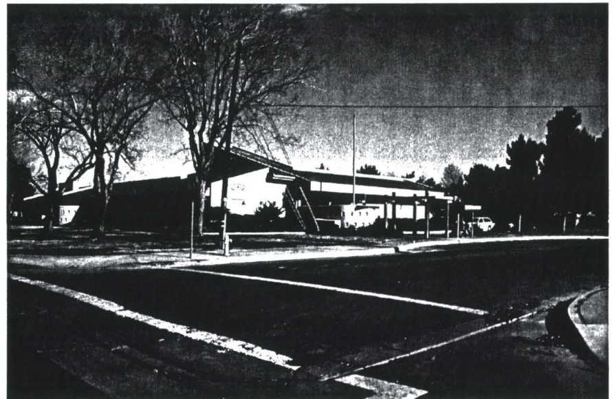
View looking northwest at the senior center / housing area.
