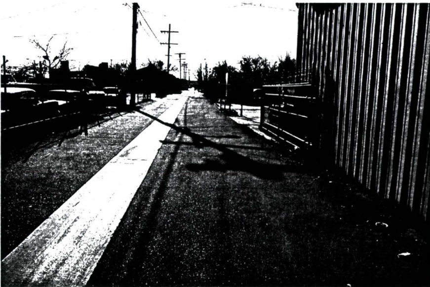
Typical view of an on-site alleyway (looking south).
