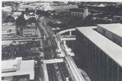
Aerial View Looking Northeast to Federal Bldg. Station
