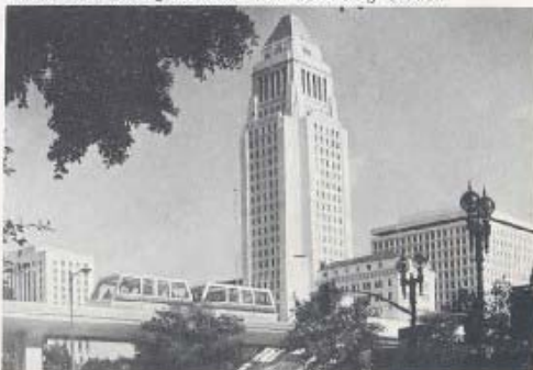
Civic Center Station Looking Northeast to City Hall
