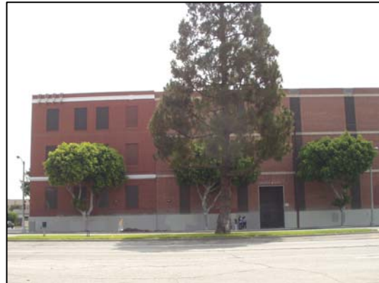
Figure 6.14: Pacific Bell new building at the east side of Vermont Ave
