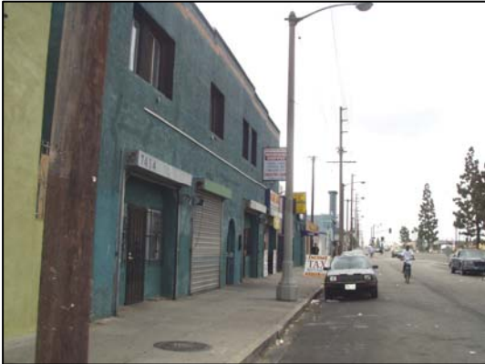
Figure 6.11: Vacant Stores at east Vermont Ave., facing south
