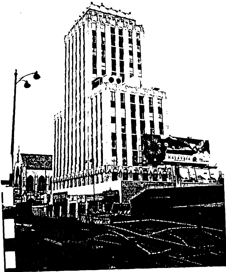
1 RE PROFESSIONAL BLDG.
