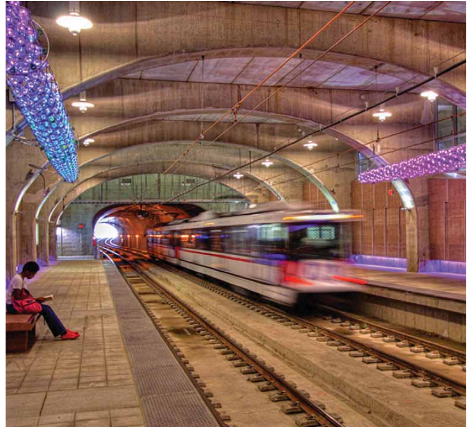
Art light element within Light Rail Station
