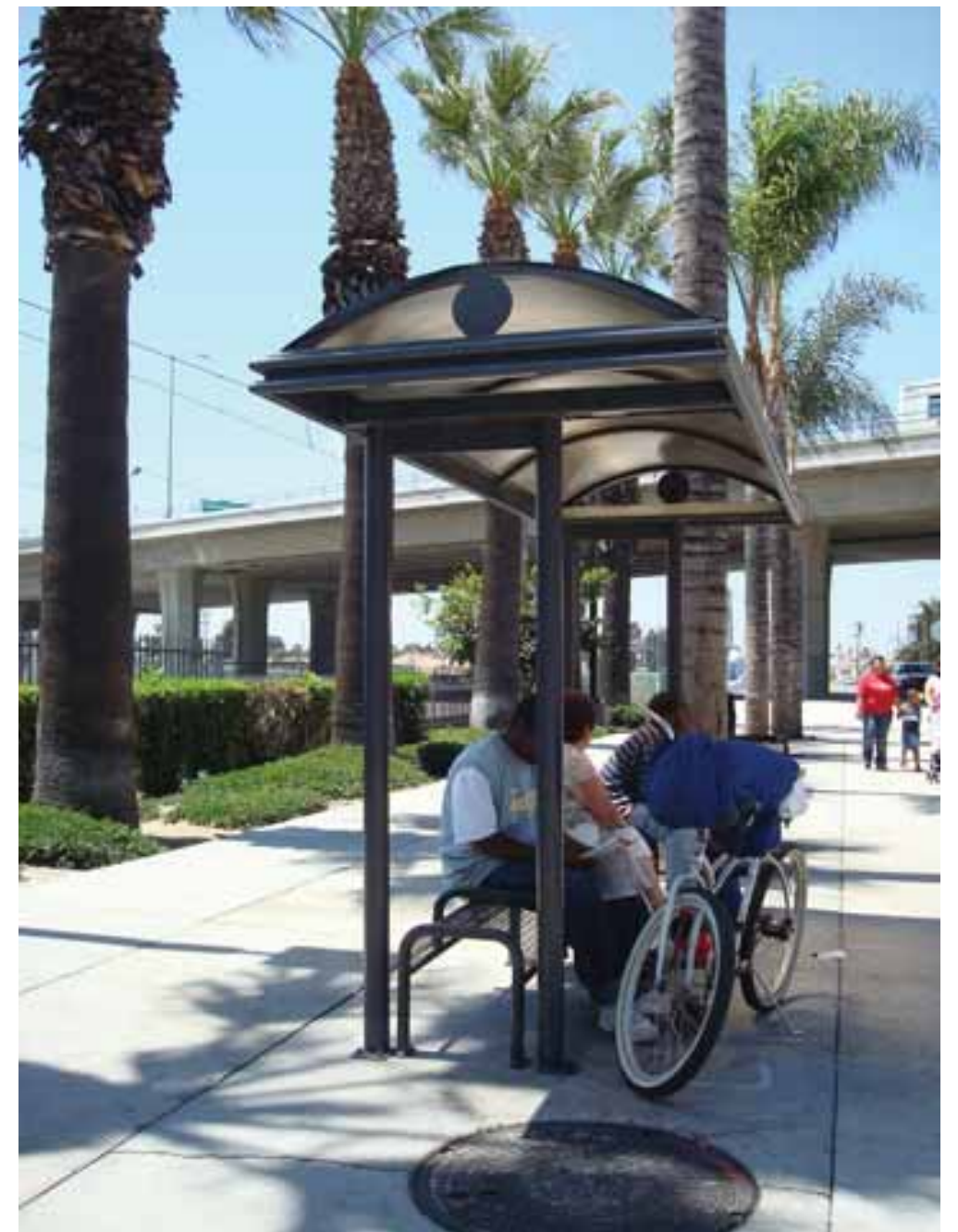
Rosa Parks Existing East Bus Kiosk
