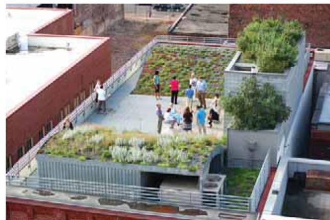
Sustainable Green Roof
