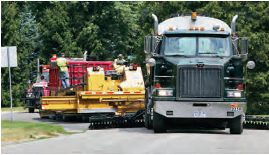
Strategies for maintaining existing assets are an integral part of transportation agencies' long-term preservation programs.
