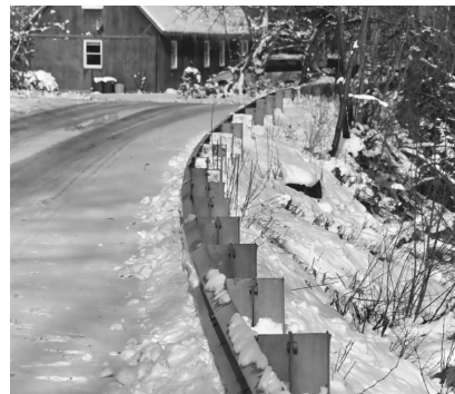
New Hampshire used NCHRP research to make guardrails safer.
