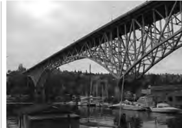
The Aurora Avenue Bridge in Seattle was seismically retrofitted with base isolation bearings. (Image courtesy of WSDOT)
