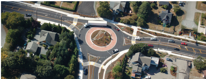
Roundabouts, which help increase safety and reduce congestion, are becoming more common in the United States through the implementation of NCHRP Project 03-65.
