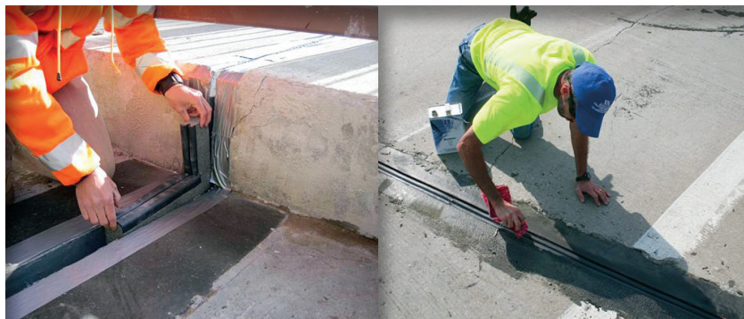
Step-by-step photos in the guidelines demonstrate the installation of several types of expansion joints, including this bonded joint seal.
