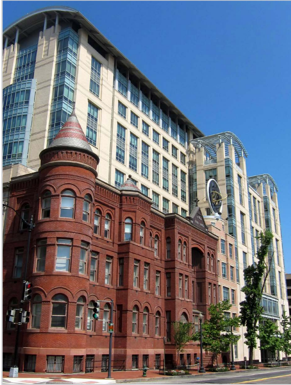
TRB is headquartered at the Keck Center of the National Academies, 500 Fifth St. NW, Washington, D.C.
