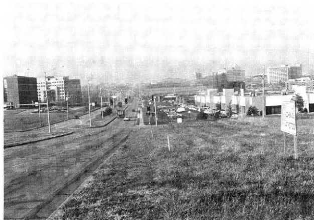
Figure 14. Four-lane divided highway with raised median used to limit strip commercial development.
