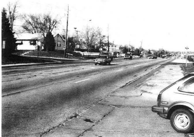
Figure 16. Inappropriate wrong-way use of intersection left-turn lane on five-lane divided highway with TWLTL.
