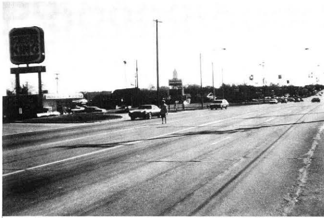
Figure 15. Problems encountered by pedestrian crossing a five-lane divided highway with TWLTL.
