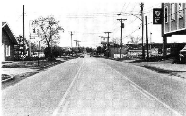
Figure 3. Three-lane divided highway with center two-way left-turn lane.
