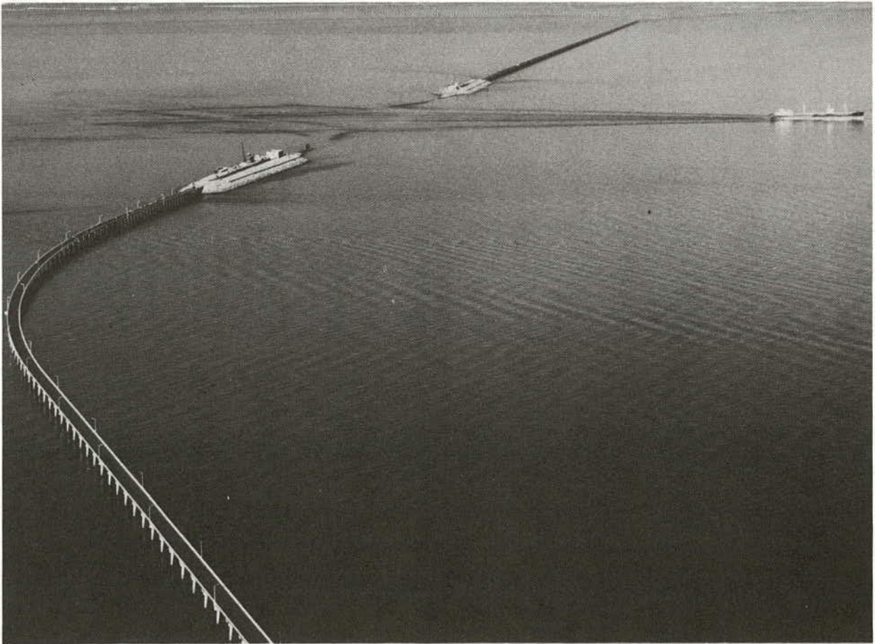
FIGURE 4 Chesapeake Bay Bridge-Tunnel.
