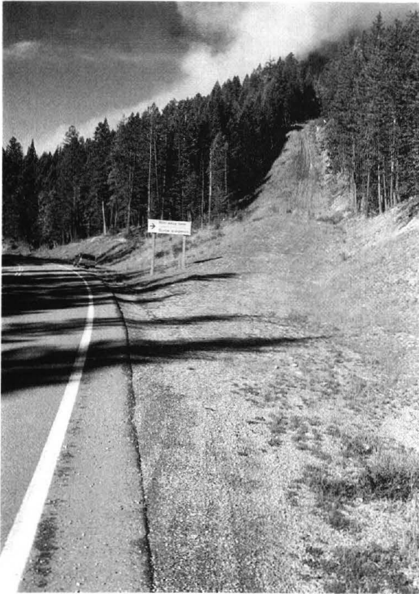
Figure 6 Example of a gravity ramp in British Columbia (possibly an old logging road).
