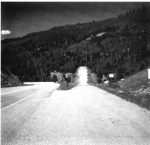
Figure 10 Ramps should be straight and should leave the roadway at the smallest angle possible.
