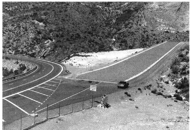
Figure 11 This Arizona site facilitates entry and use by more than one vehicle at a time. Note pavement marking to minimize parking or confusion about the main travel lane direction.
