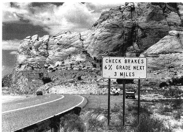
Figure 16 A brake check area created at the top of a grade in Arizona.
