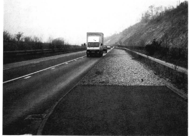
Figure 8 An early version of a gravel arrester bed along shoulder of a British motorway.
