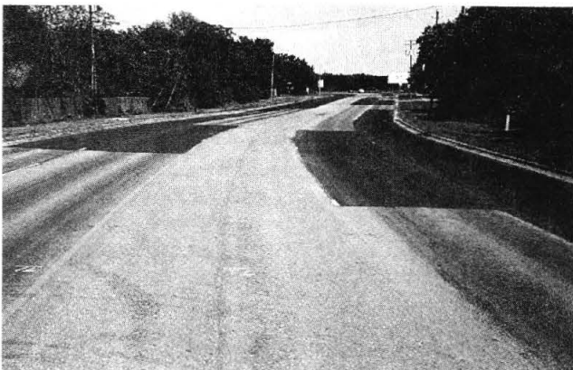
Figure 10 A patchwork surface will cause difficulty in controlling mixture design during HIPR and, therefore, may be an unsuitable candidate.
