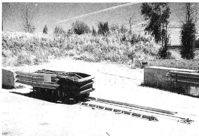
Figure 2 The GREAT system after impact. (Courtesy of Energy Absorption Systems, Inc.)
