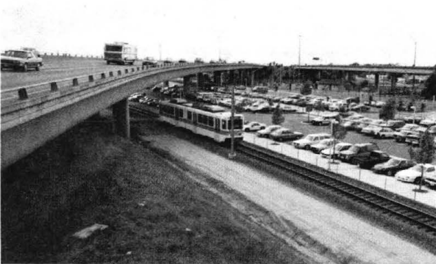
FIGURE 4 Park-and-ride lot with LRT. (Courtesy of Sacramento Regional Transit District)
