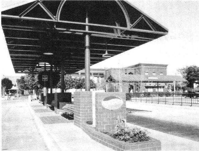
FIGURE 16 Park-and-ride lot bus station area, Fullerton, California. (Courtesy of Parsons Brinckerhoff)
