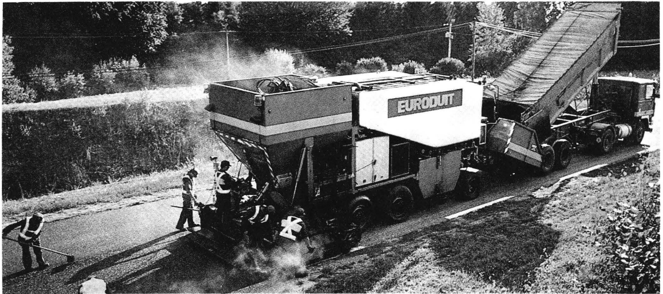
FIGURE 4 NOVACHIP paving equipment.
