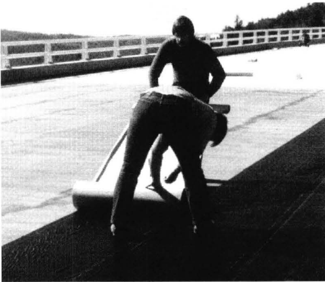
FIGURE 18 Application of a self-adhesive preformed membrane. (Courtesy of Vermont Agency of Transportation)
