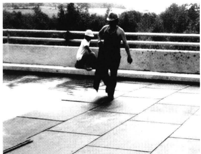
FIGURE 24 Protection boards applied over a rubberized asphalt membrane.
