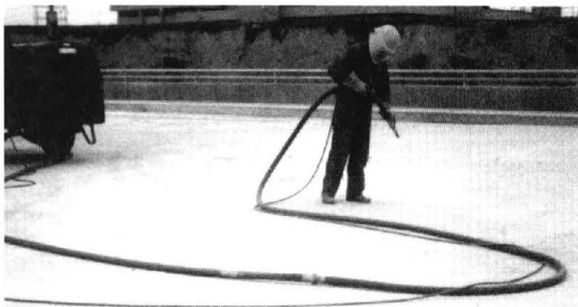
FIGURE 13 Sand blasting a bridge deck prior to waterproofing.
