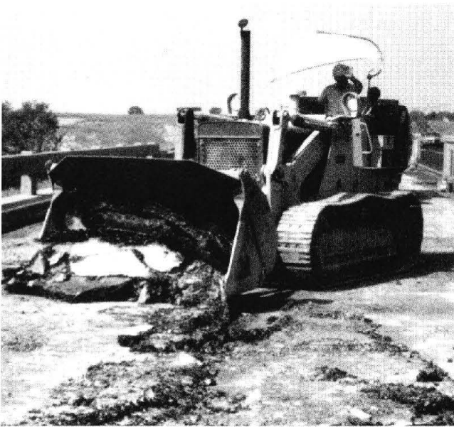
FIGURE 29 Use of a bucket to remove surfacing and poorly bonded membrane.
