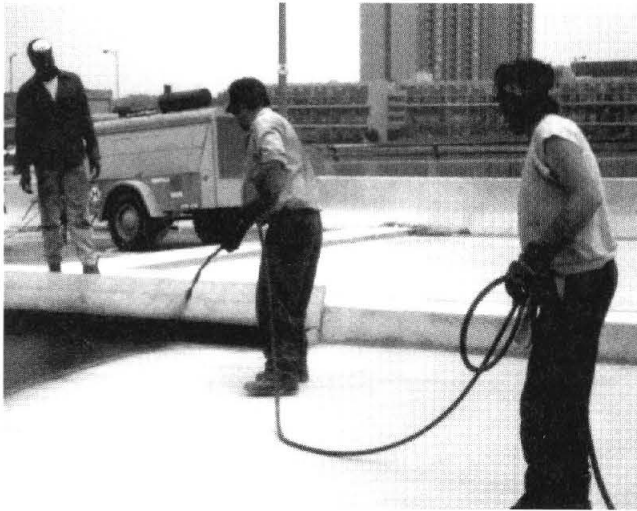
FIGURE 14 Application of an asphalt emulsion primer using a spray.
