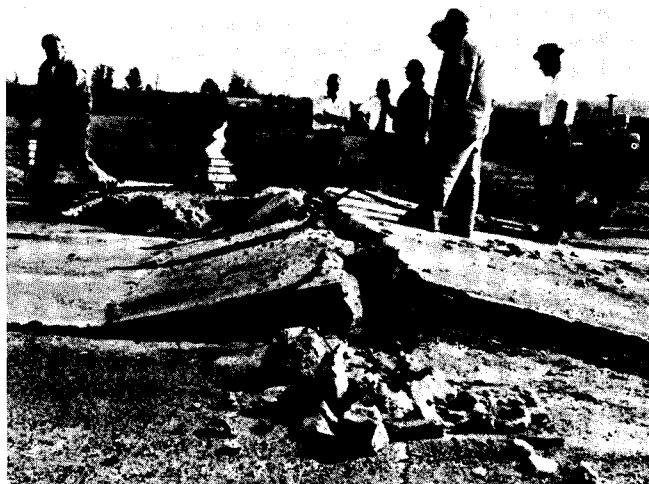
FIGURE A-8 Blowup of portland cement concrete pavement (15).
