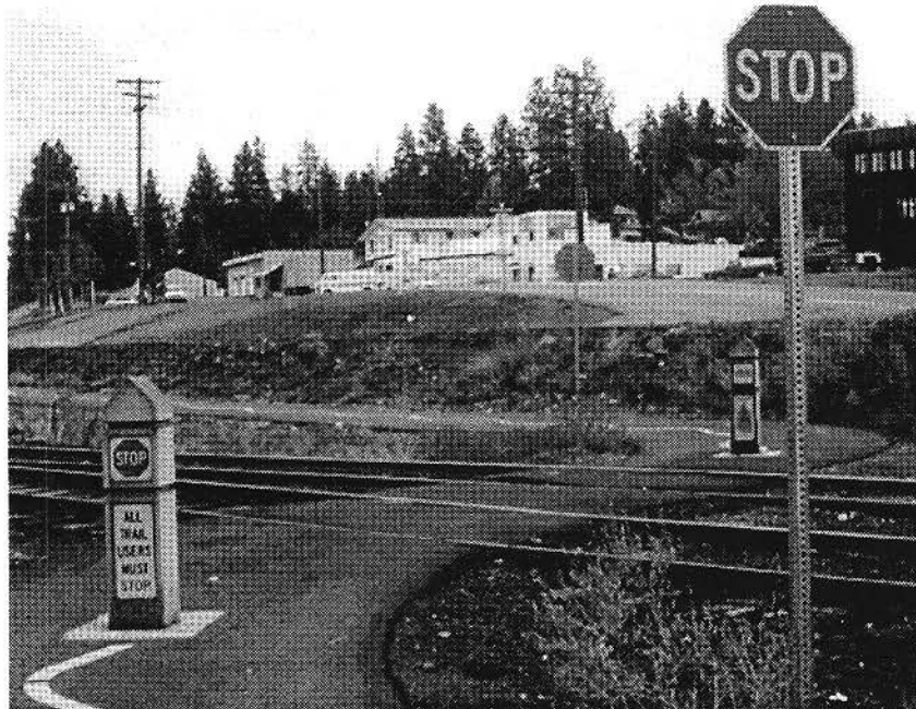
FIGURE 16 Relocated bike path to elevate bad-angle crossing.
