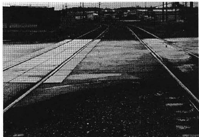
FIGURE 23 Multiple tracks in a crossing with different elevations.
