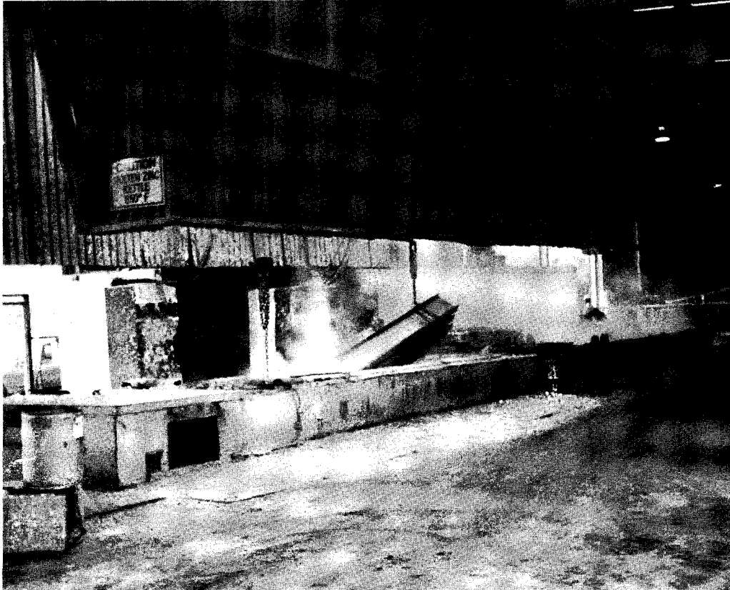
FIGURE 10 Galvanizing dip tank.
