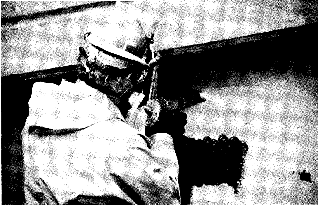
FIGURE 19 Ultrahigh pressure water jetting.
