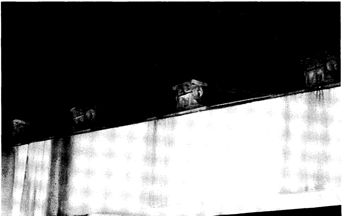
FIGURE 11 Installed galvanized bearing.
