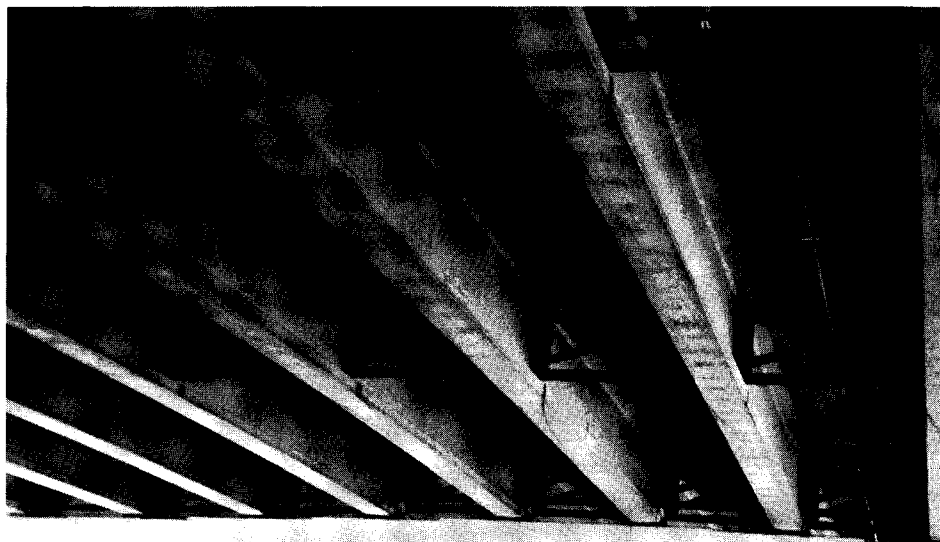
FIGURE 14 Weathering steel diaphragms with prestressed beams.
